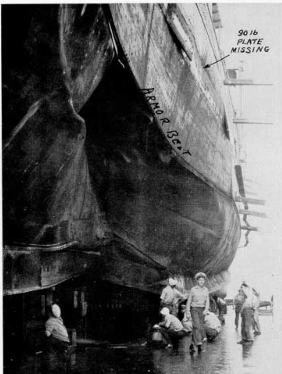
Photo 2: USS CHESTER - View of torpedo hole from dry dock floor.
