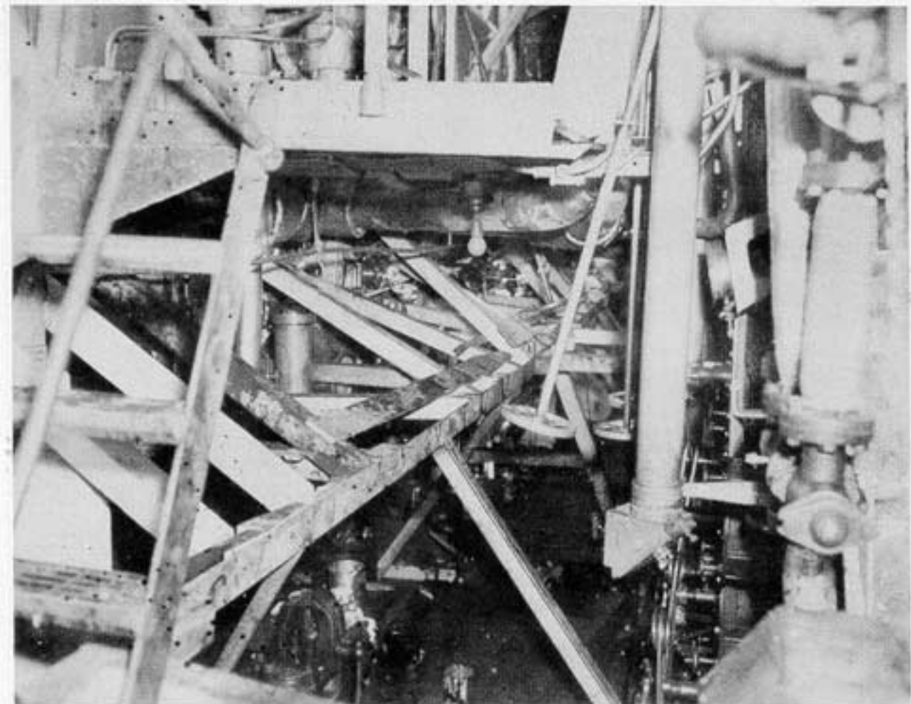
Photo 13: USS CHESTER - No. 2 fireroom from starboard gratings showing part of the upper course of shoring on bulkhead 64.
