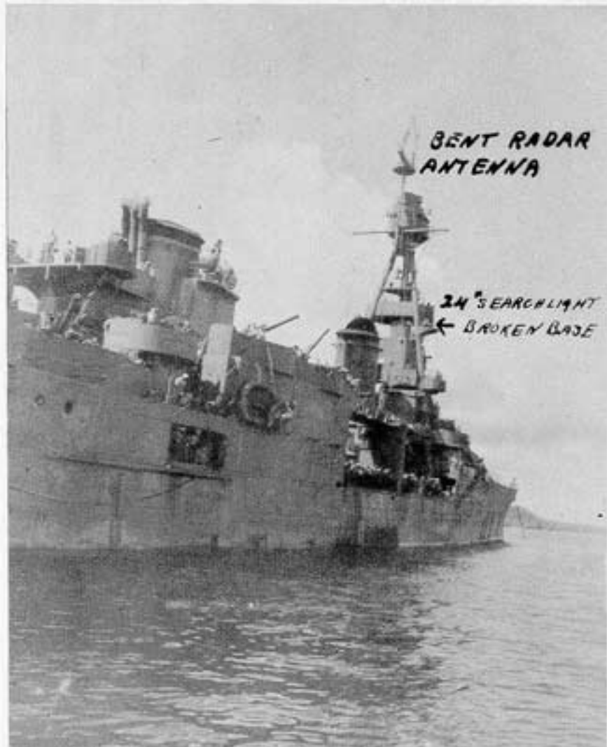
Photo 1: USS CHESTER - General view from starboard quarter showing armor plate missing above hole, broken searchlight, bent radar and damaged life rafts.
