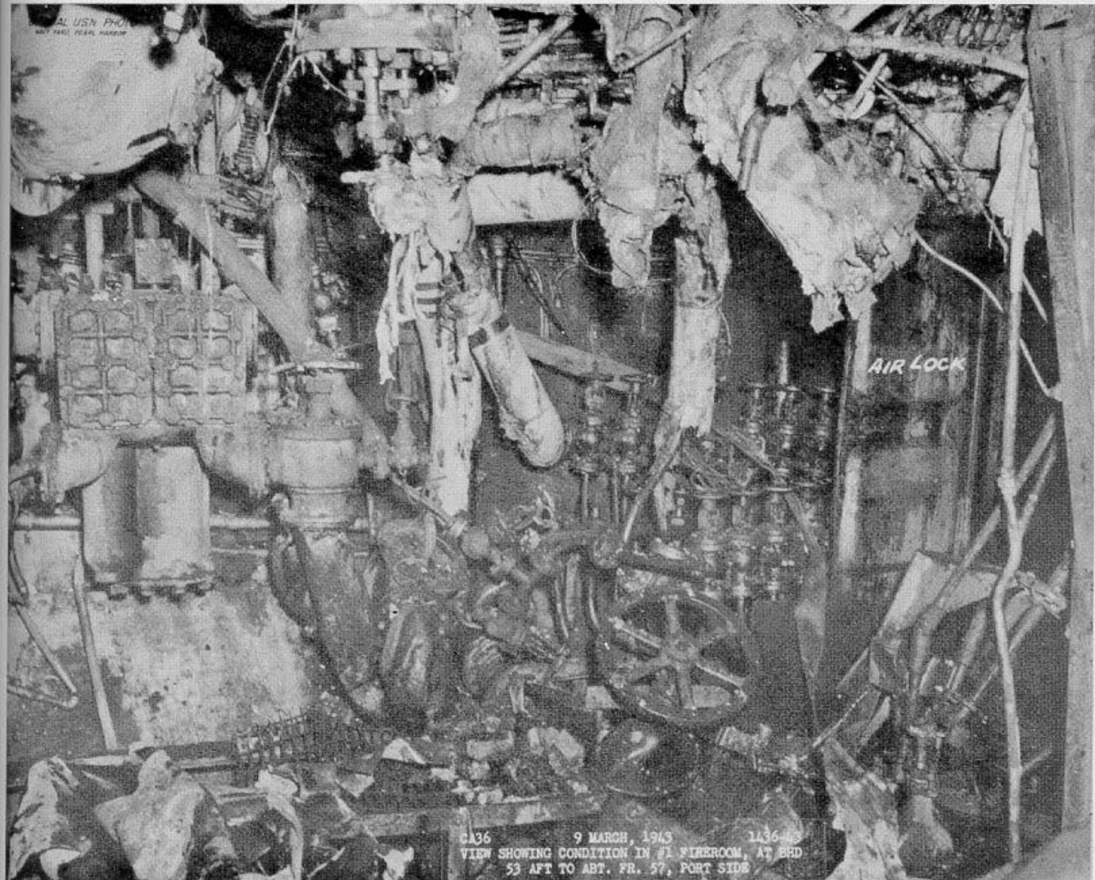
Photo No.25: USS MINNEAPOLIS - Port side No. 1 fireroom.
